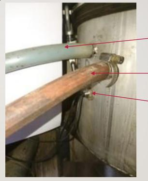
Condensate pipe of condensate pump
